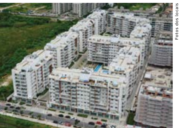
FRAMES RESIDENCE RECREIO DOS BANDEIRANTES
